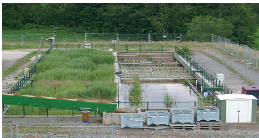
Fig. 9.17 Wismut-designed mine water treatment system with rooted plants receiving water from the right side for treatment. On the right side, in the open water, Boojum recommended installing curtains for biofilm formation and floating cattail islands to address fine iron particles. In the foreground some cattail islands grew well, but others were plagued leaf lice. The light blue buckets were installed to provide a flow-through system for Chara . Growth data were used to derive design criteria for scale-up
